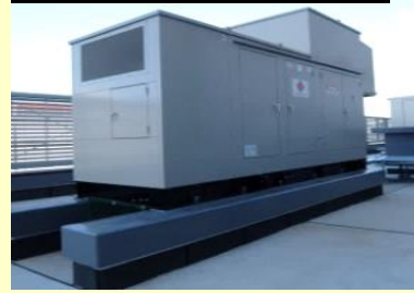
Emergency power generator
