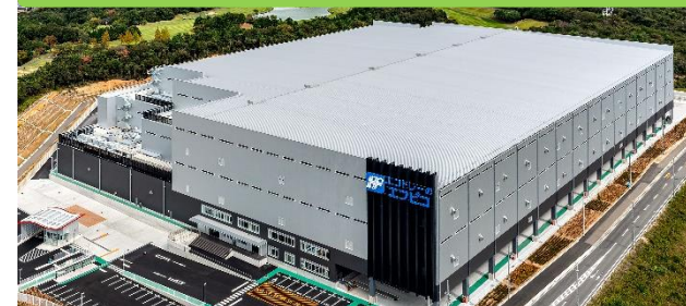
System for Fukuyama Recycling Plant Commencement of operation planned in the summer of 2023
