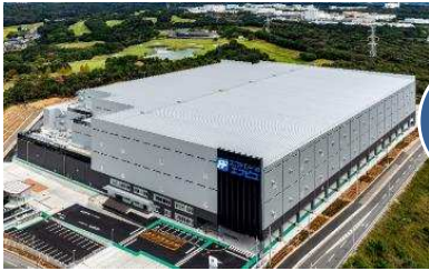
Kansai Plant and Kansai Hub Center Commencement of operation: January 2023 Investment: 26,670 million yen Total floor area: 79,883.65 m 2
