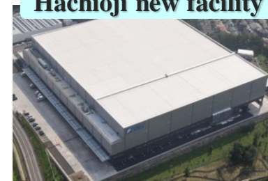
DC in Nov. 2014 and PC in Feb. 2015, Second phase construction was finished in Sep. 2015
