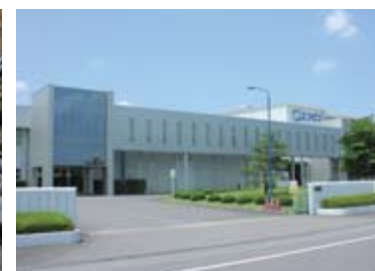
Kanto Shimodate Plant
