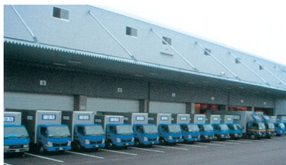
Twenty-three trucks can park at the same time in the truck berths
