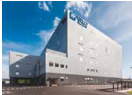
Kansai Distribution Center / I-Logic Kansai Picking Center (inaugurated in October 2013)
