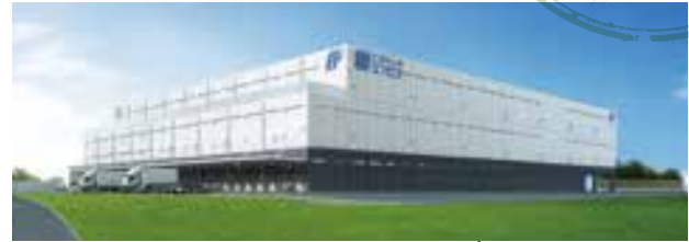
Hachioji Distribution Center (inauguration due in September 2014)
