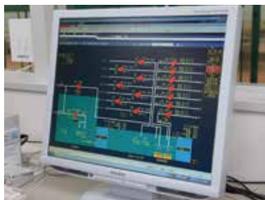
Display Monitor of the Centralized Management System
