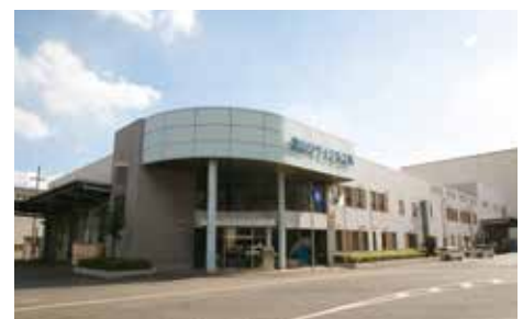
Fukuyama Recycling Plant
