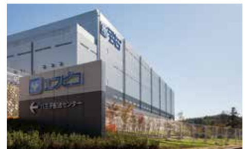
Hachioji Distribution Center
