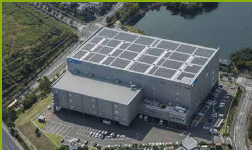
The Kansai Distribution Center is equipped with solar panels on its roof.
