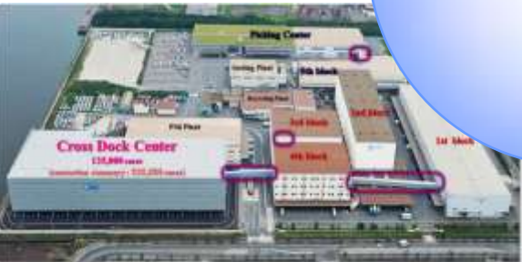
Fukuyama Cross Dock Center Started operation in Aug.2014
