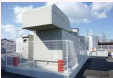
Chubu Distribution Center II
