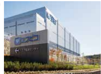
Hachioji Distribution Center
