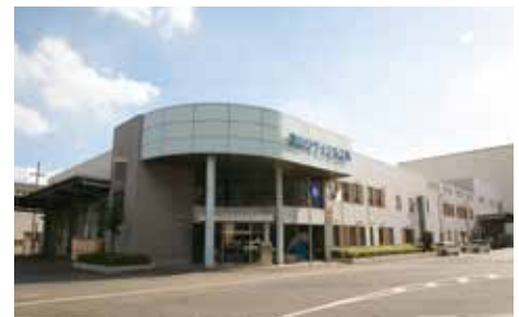
Fukuyama Recycling Plant
