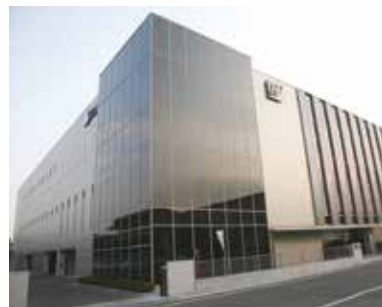
Fukuyama Headquarters (Fukuyama-shi, Hiroshima)
