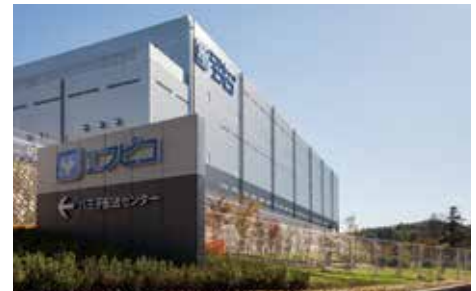
Hachioji Distribution Center
