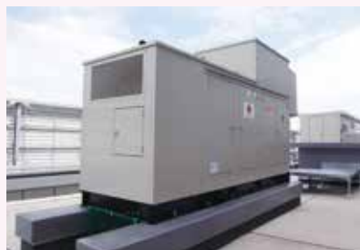
Hachioji Distribution Center
