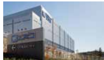
Hachioji Distribution Center
