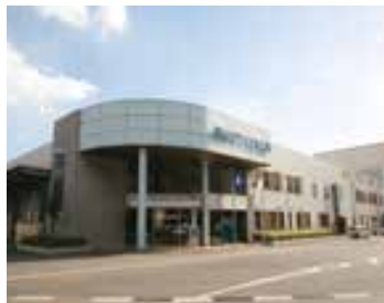
Fukuyama Recycling Plant
