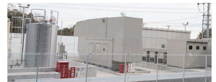
Power supply in emergencies: Emergency power generation equipment installed at our logistics facilities capable of supplying power for 72 hours.
